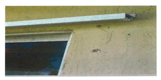
2) Install one side angle and level from the end of the top track.
