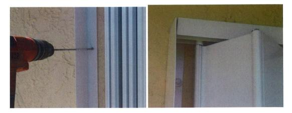
6) Make sure accordion stack is completely open and tightly stacked before attaching the accordion starter to the angle with # 10 x 3/4 tech screws.
