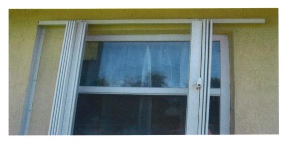
4) Install bottom track with ¼" clearance between the shutter blades and bottom track.
