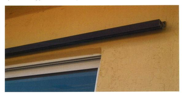
3.) Install one side angle and level from the end of the top track.
