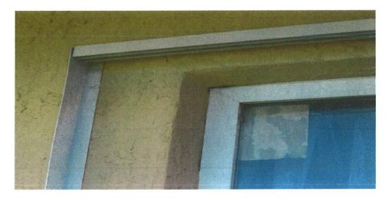
3) Install blades by sliding wheels in through the open end, opposite the angle.
