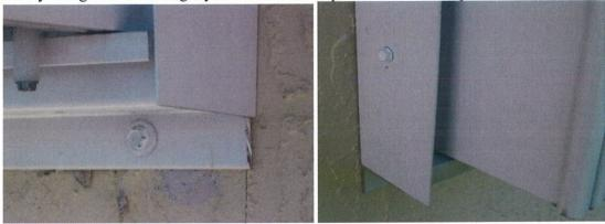
Below: Application with 1x1 side angles. The starter can be installed on the inside or on the outside of the angle.
